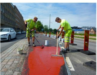
By the development of our PlastiRoute® hc (hot climate) we have extended our product portfolio. Especially in challenging climate areas PlastiRoute® hc is used successfully and can be delivered in different material classes depending on application technique.
